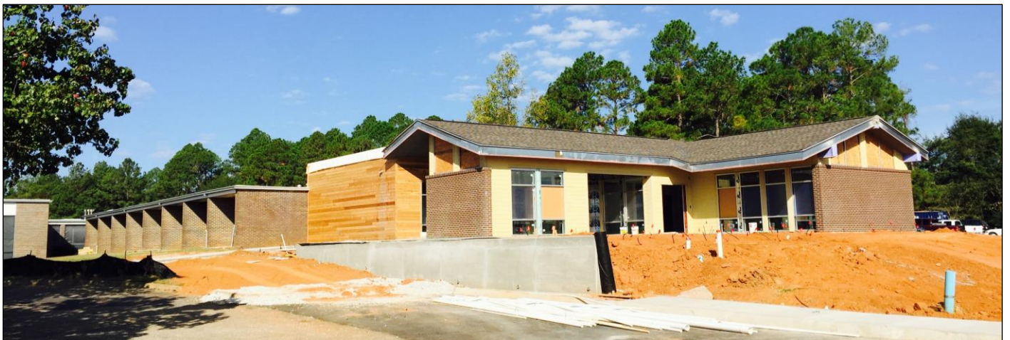
The Rehab Inn Nearing Exterior Completion
